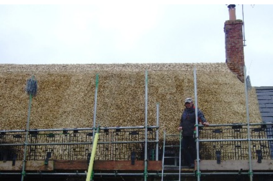
Dan Quartermain re-thatching a cottage at Tysoe, Warwickshire in November
