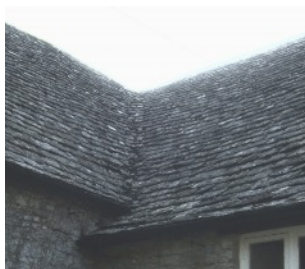
A swept valley- Anchor Cottage Coln St Denys
