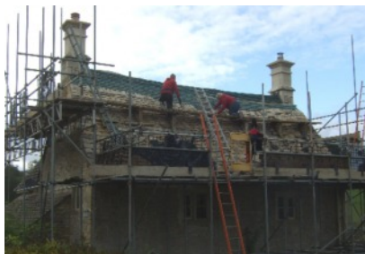
Martin and Hannah Jewell and the team from Hill and Valley Builders reroofing Blakemoor Cottage Chedworth in the autumn..
